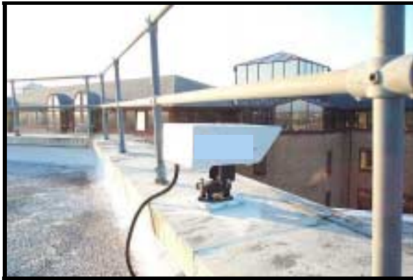
Figure 2.6: Parapet/Ledge Mounting (using JMP only)
